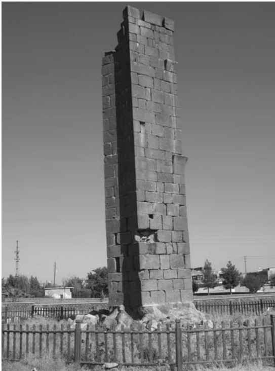
Fig. 2.7.4 Surviving pier of the Octagon
